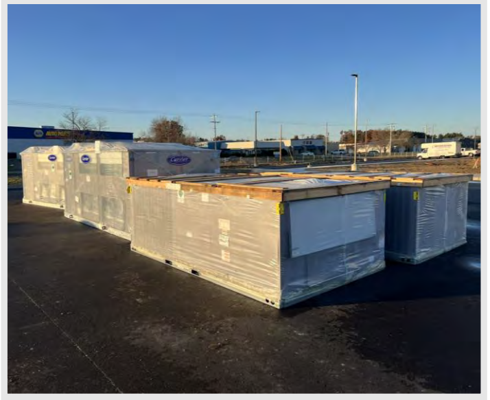
The mechanical Roof Top Units (RTUs) are being staged on site in preparation for setting them in place in the coming weeks.
