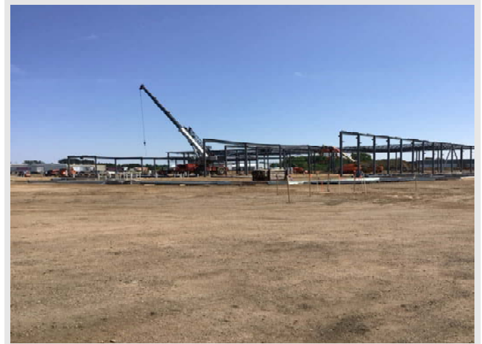
One week of structural steel progress
