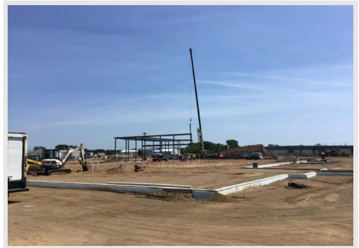
The start of structural steel as of 06/01/2023
