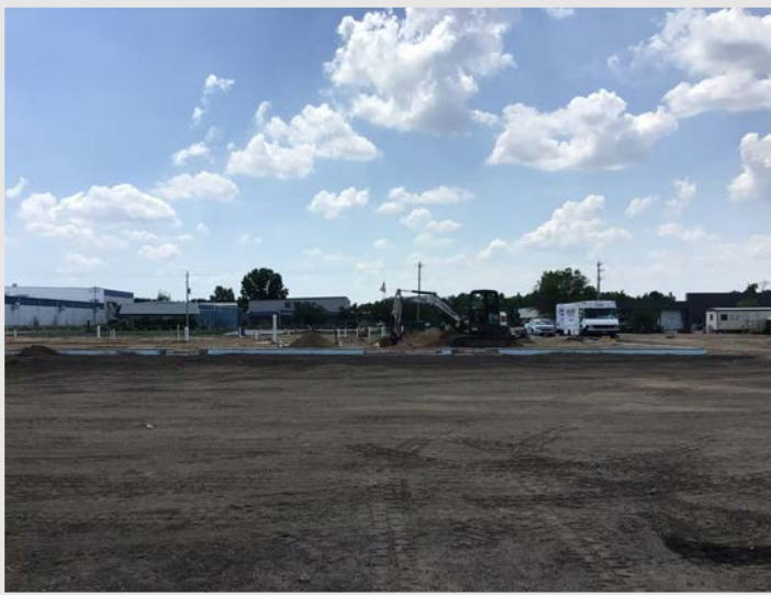
Underground Plumbing being installed ahead of steel erection
